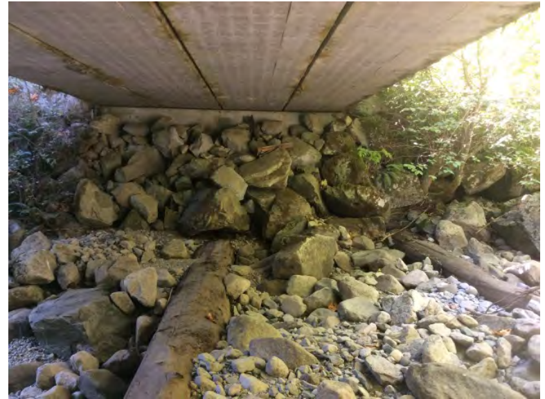
Right Bank Abutment when facing downstream
