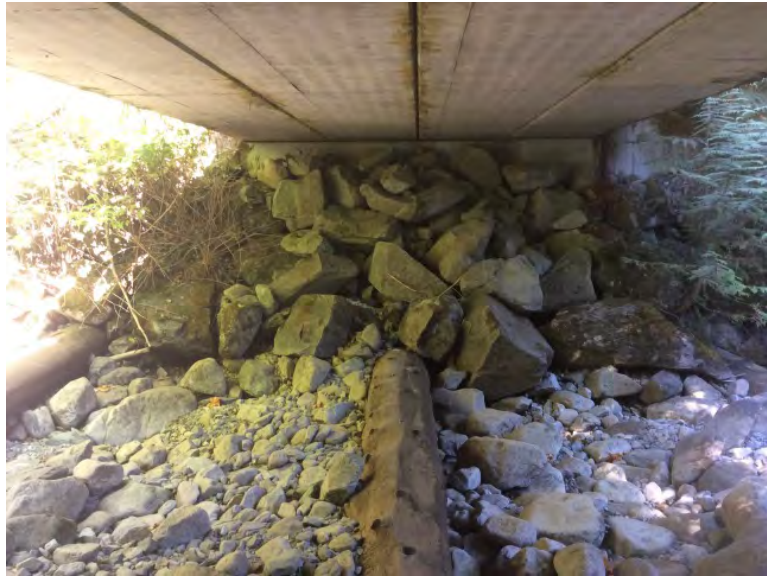
Left Bank Abutment when facing downstream
