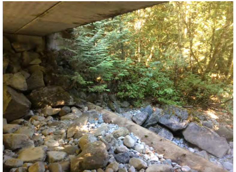
Left Bank Abutment when facing downstream
