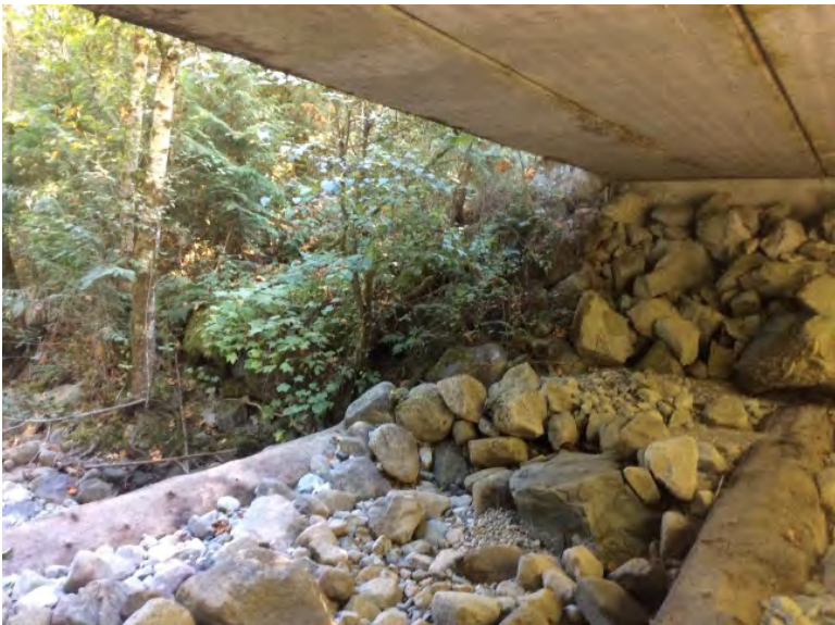
Right Bank Abutment when facing downstream
